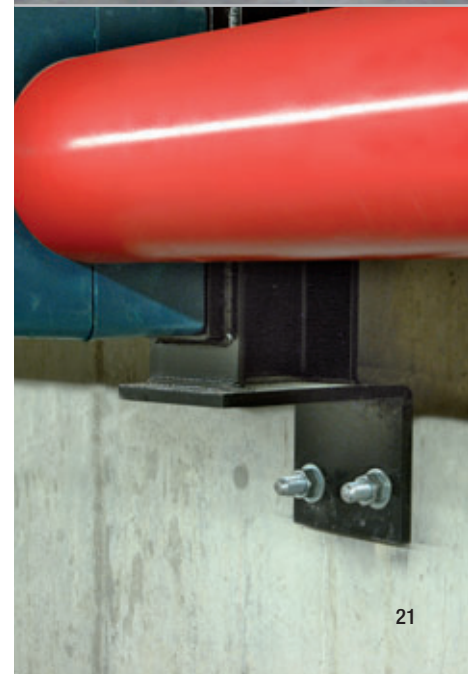
Apply recommended fastening torque with a calibrated torque-wrench
