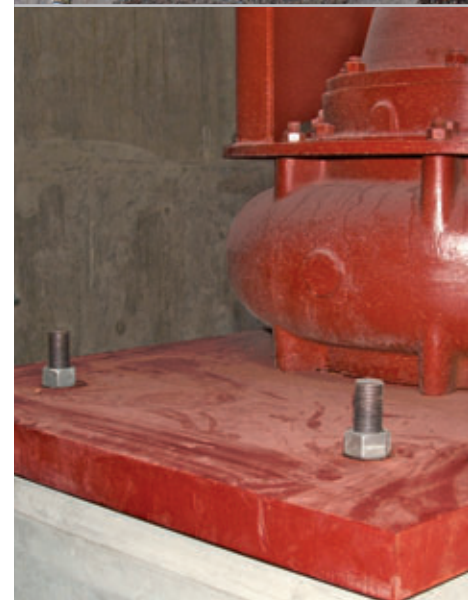
Attach fixture and apply the recommended fastening torque with a calibrated torque wrench
